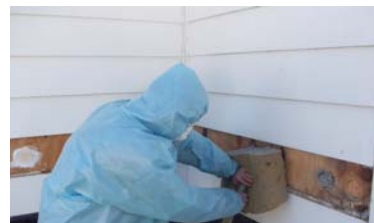
Weatherization Crew insulating a home
